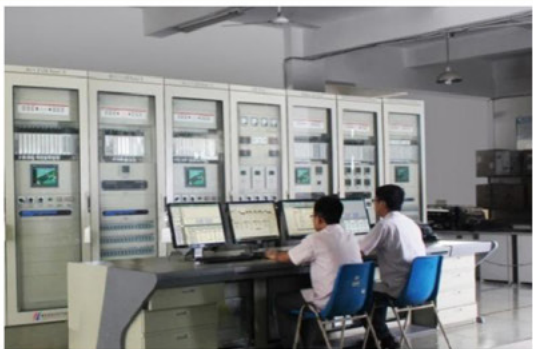
监控保护及直流系统 Monitoring, protection relay and DC
